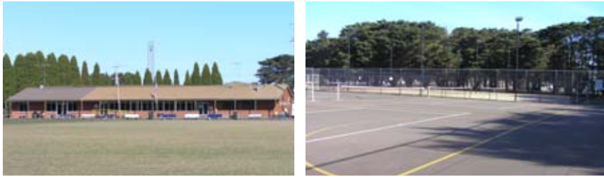
Football ground, clubrooms and tennis courts at the Lara Recreation Reserve
