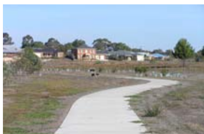
Recently completed shared path along Serendip Creek which will eventually connect the town centre to the You Yangs.
